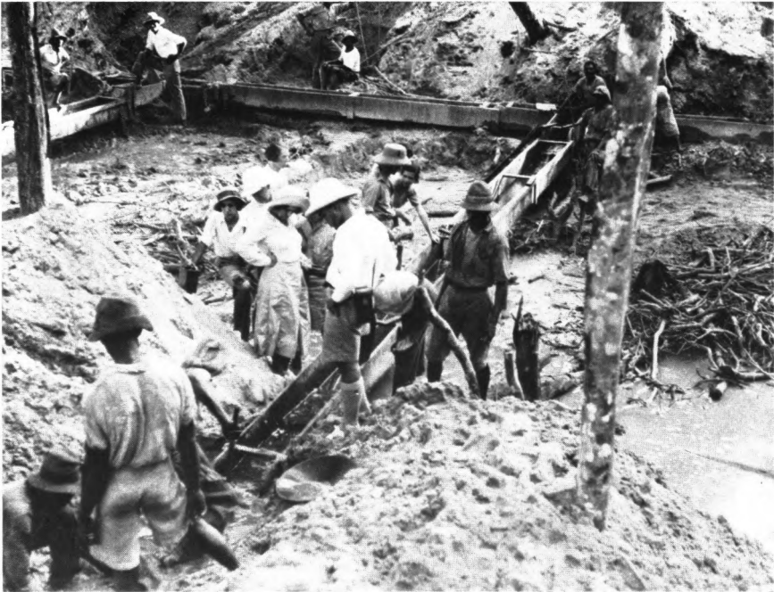
62 Washing gold-bearing gravel in the Belgian Congo in the 1920s by fairly primitive methods more typical of the nineteenth century
